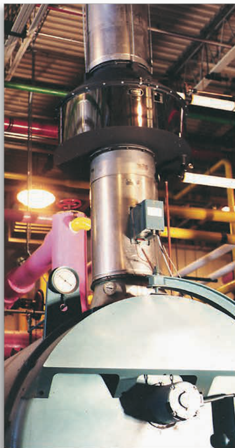
Printing Facility, Lomira, Wisconsin (2) Model: FCR-112C16ALS each Recovering Btu from a 500 BHP steam boiler; Reducing 400°F @ 4205 SCFM to 252; Raising 34.5 gpm boiler feedwater entering at 120°F to 164°F.
